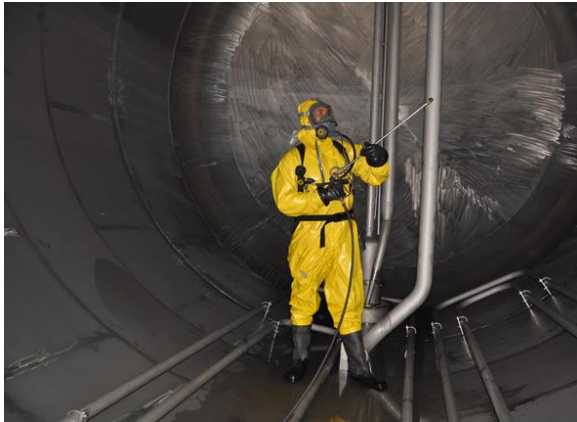
Cleaning of fuel/chemical tanks
